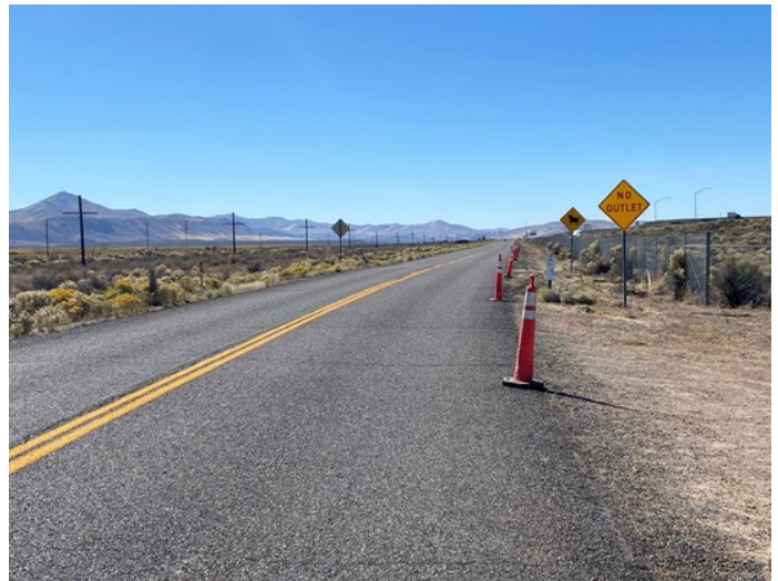
Stretch of W. Idaho St. on the way to the Trail Center with no shoulder. This road ends at I-80 exit 303.
